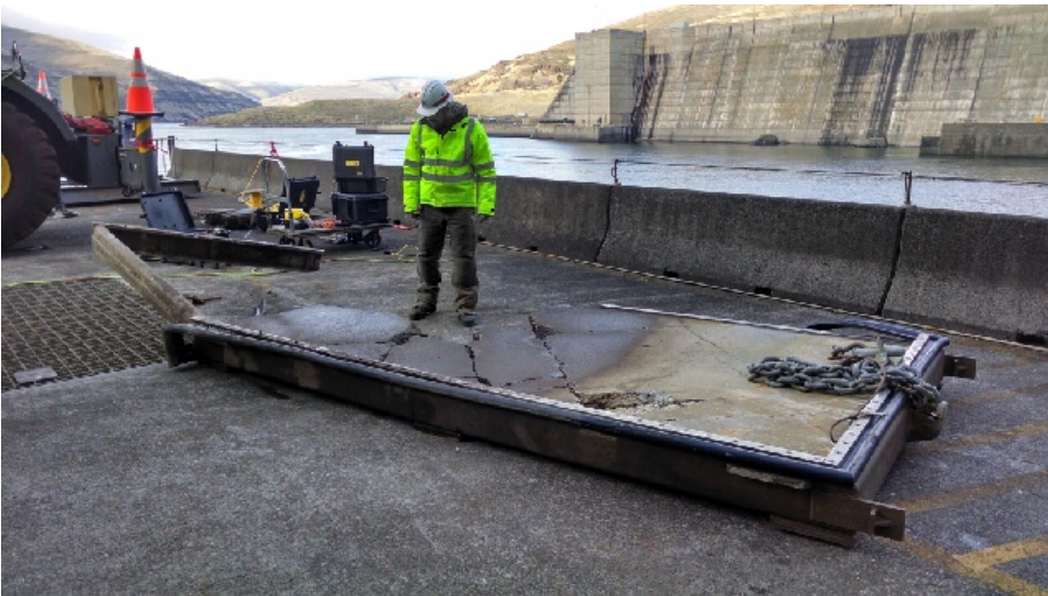
Picture 1. NPE 3 after it was removed January 2015.
